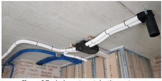
Figure 6 Typical apartment ducting system.
