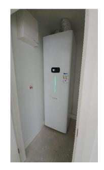
Figure 1 Typical Exhaust Air Heat Pump (EAHP) Unit.
