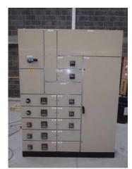
Figure 8 Typical Form 4 main distribution board.
